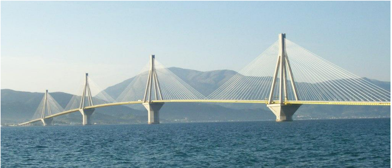
View of the bridge from the University of Patras.
